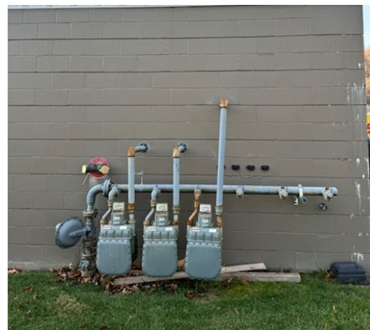
Exterior Gas Main Shutoff
